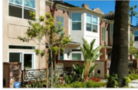
YARD, FORECOURTS, AND BUILDING ENTRIES
