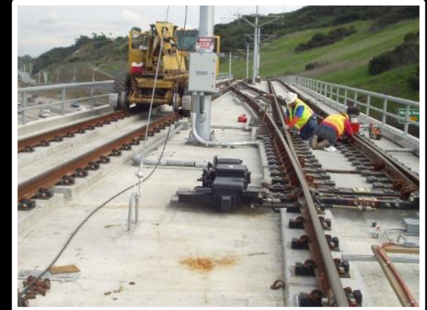
Track Work and Systems
