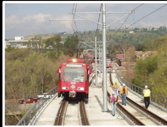
Stations/Parking, Communications and Security
