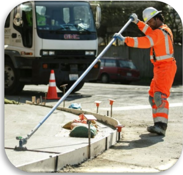
Construct Missing Sidewalks
